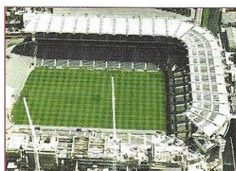
2000 THE HOGAN STAND IS UNDERWAY
