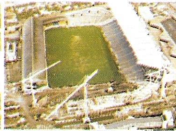
1998 CANAL END CONSTRUCTION
