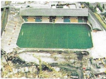
1993 CUSACK STAND DEMOLISHED
