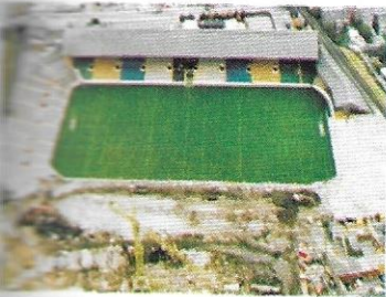
1998 SACK STAND DEMOLISHED
