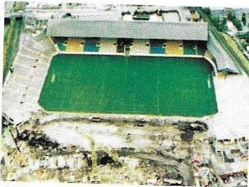
1993 CUSACK STAND DEMOLISHED
