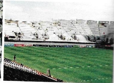
2004 HILL 16 / NALLY STAND CONSTRUCTION
