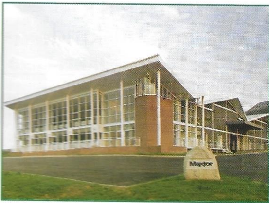
Industrial Administrative Unit, Boghall Road, Bray.
