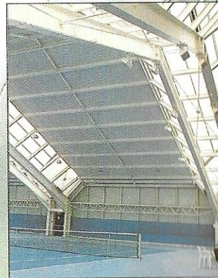
Roof Panels and Translucent Sheetting
