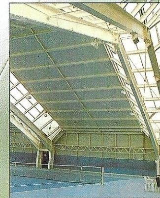
Roof Panels and Translucent Sheetling
